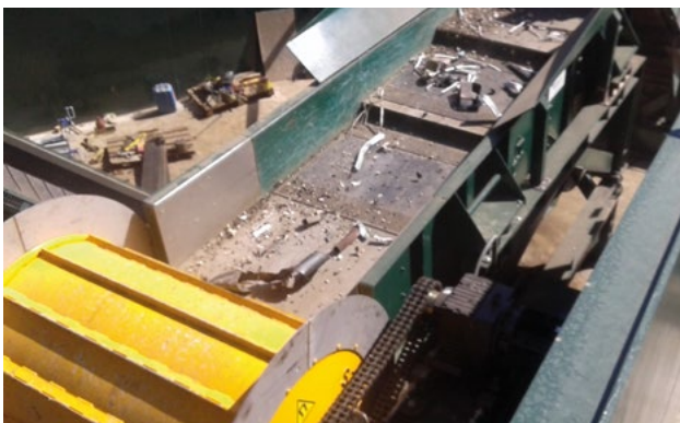
FEEDER TO MAGNETIC DRUM SEPARATOR
